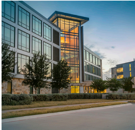
Drone Survey Image Date Captured: 9/2018
